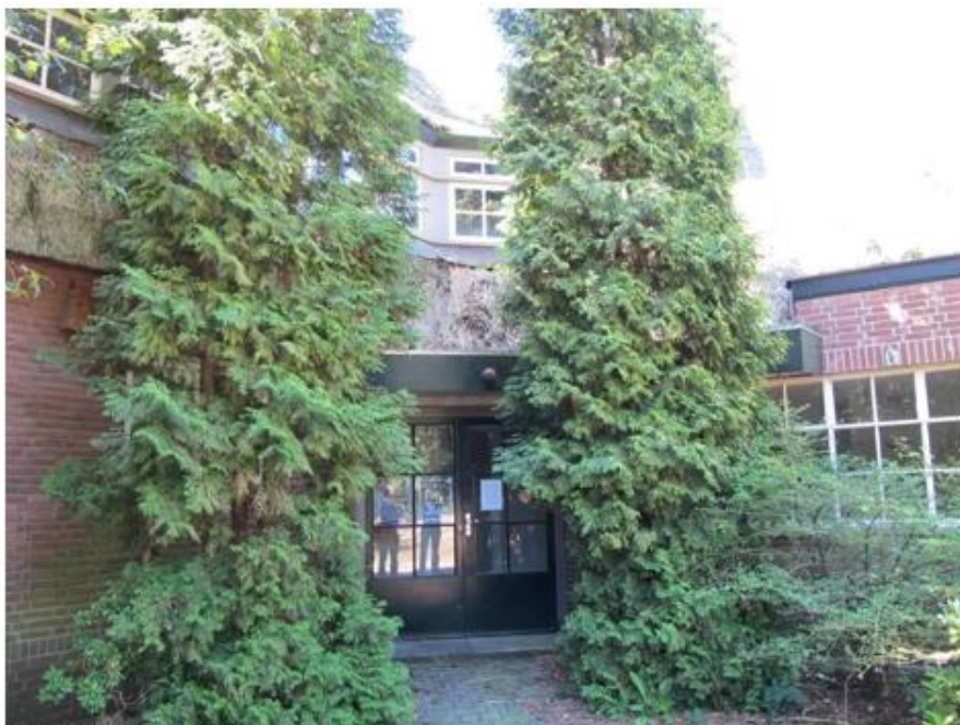
Entree in de noordgevel. (MAB, 2011)
