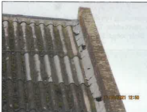
Gaten langs dakrand/loodslabbe
