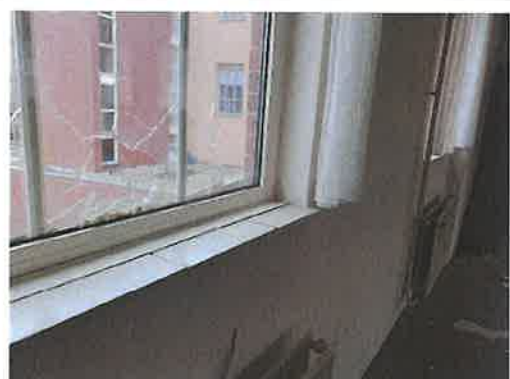
Beglazing (in rubber) en vensterbanken
